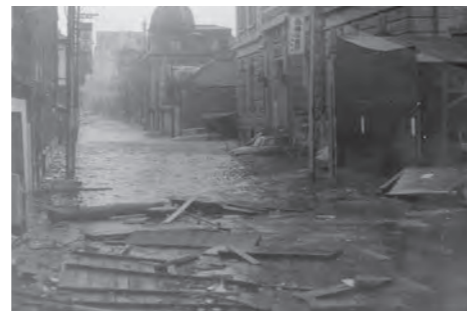
Second Muroto Typhoon, September 16, 1961
